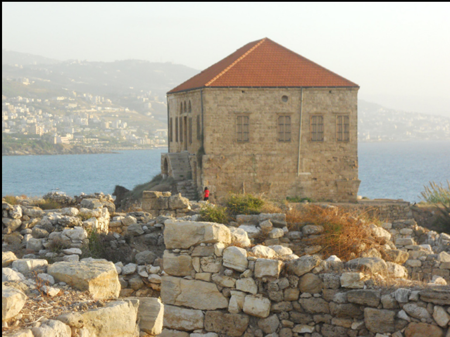
134 typical Lebanese house
